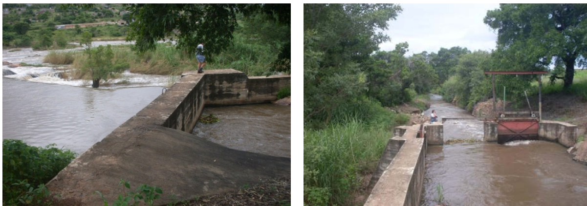
Figure 9.5: Kaapmuiden weir and inlet to the Van Graan Canal
